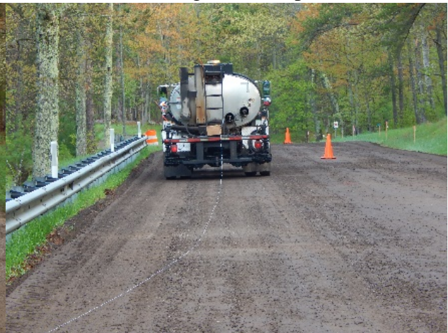
(f) Boundary control of the pavement
