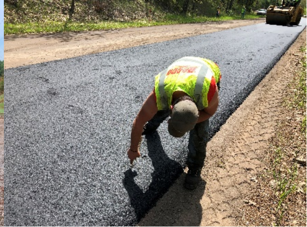
(b) Leveling layer thickness control
