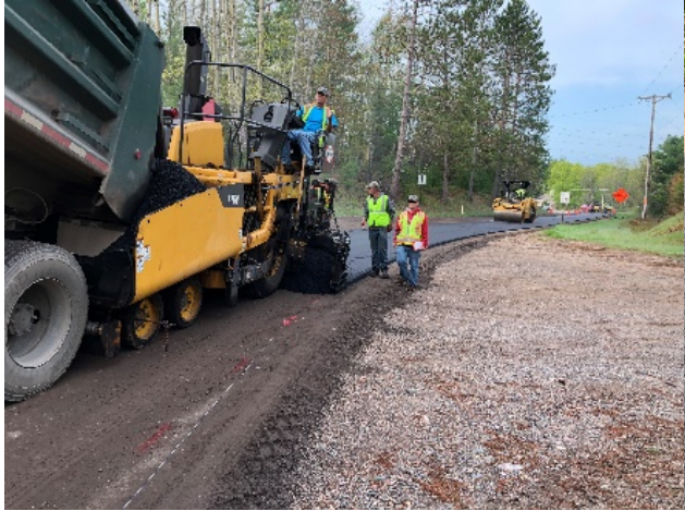
(a) Leveling layer compaction
