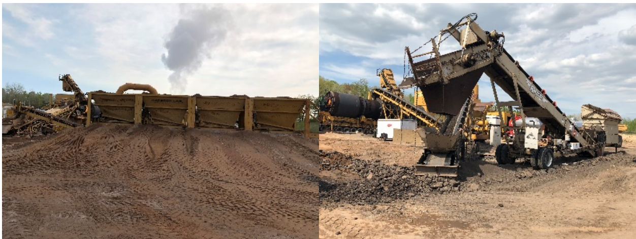
(a) Aggregate feeding system
