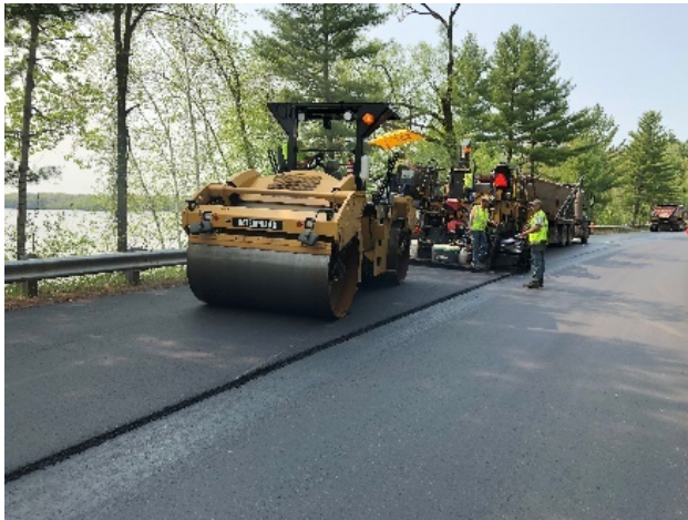
(e) Surface layer compaction
