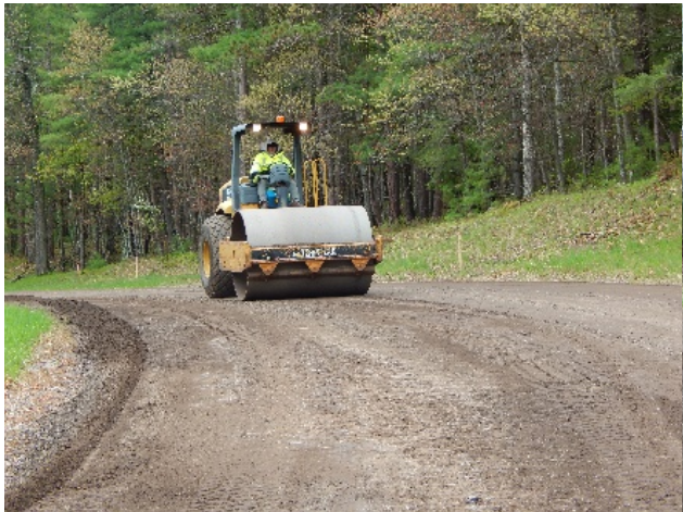
(c) Compaction of the old surface layer
