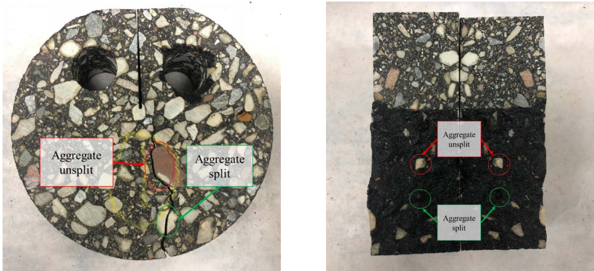
(a) The surface view of the cracking path
