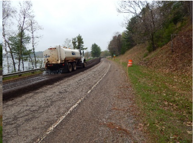
(b) Water spray after milling
