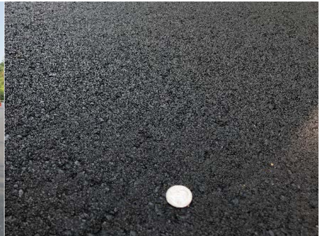
(f) Final pavement condition
