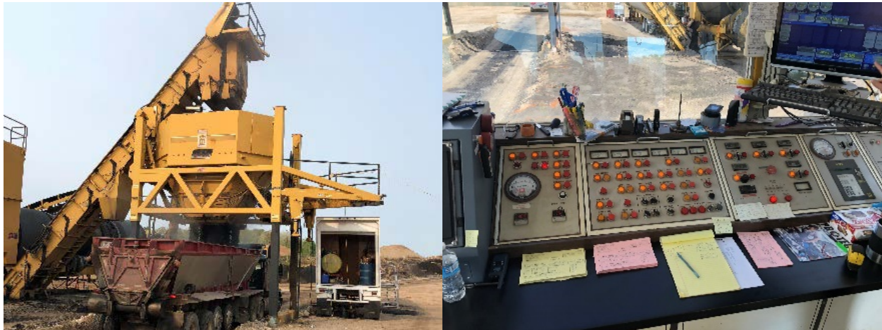
(e) Mixture storage silo
