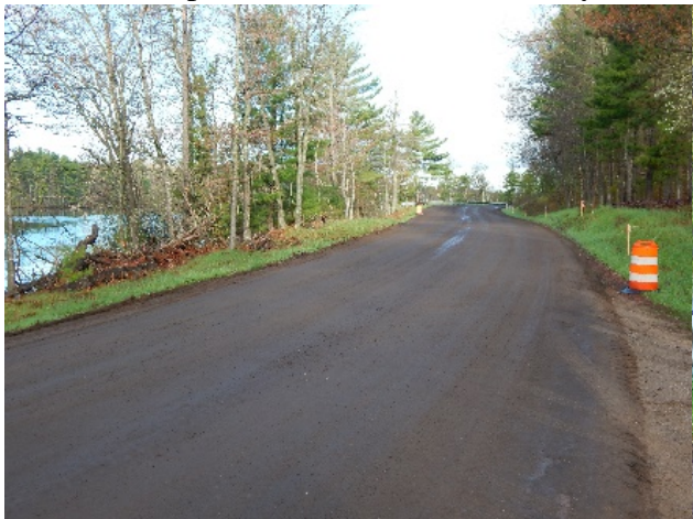
(e) Old surface layer as the base layer
