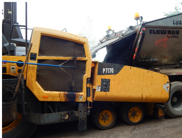
Figure 1-2 Paving operation – same as the conventional asphalt pavement
