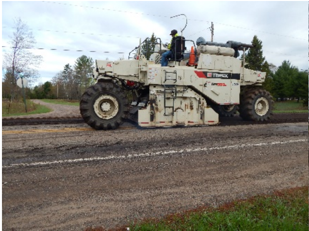
(a) Surface layer milling
